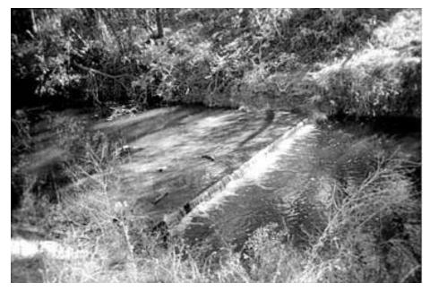
Photo #3. Drop structure (about half a foot) on Arroyo Del Valle at the end of Corte Monterey near Bernal and 680 in Pleasanton, 50 yards upstream from the Arroyo De La Laguna. At low to moderate flow this structure might block fish passage due to the flat apron above the drop and a slot might need to be cut in the concrete.
