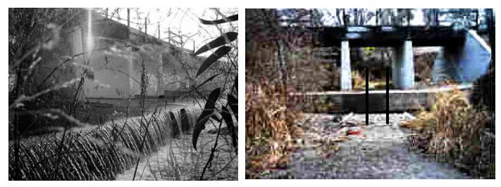
Photo #1. Drop structure (three foot) on Arroyo Mocho at Stanley and Murrieta Blvds at the old Southern Pacific railroad bridge in Livermore. A slot as shown needs to be cut in the concrete to allow fish passage.
