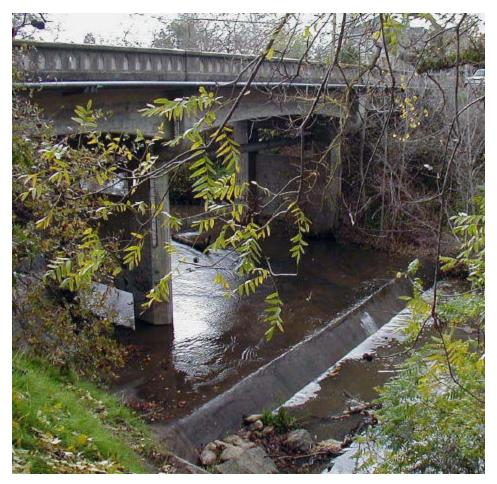
Photo #5. Drop structure (a few feet) on Arroyo Del Valle where Division Street crosses in Pleasanton. At low to moderate flows this structure blocks fish passage due to the flat apron above the drop.
